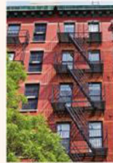
6 a fire escape
